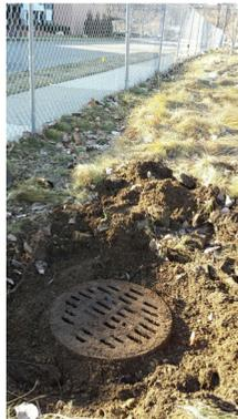
Stormwater is proposed to outlet to an existing catch basin R-37, which is shown connecting to a 12” public storm line in Nielsen Court. This storm line and catch basin do not show up in the City’s GIS inventory of public storm infrastructure. Has this “existing” storm line and catch basin been verified?
